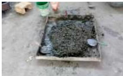
Mixing of Concrete
